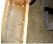
You need to notch the riser to fit the wall just like the original base.
