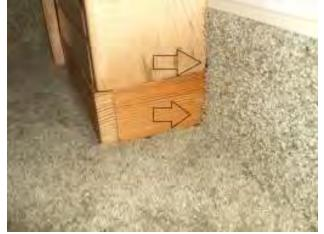
Now you can stain the bottom risers, if you want to, to match and let dry. After the bottom riser has dried, you can now move the table to be reattached to the side wall. Route the electrical cords thru there holes to be reinstalled later. Pull out the table top so you can reattach the holding screws. Set the table frame to fit the wide L braces and adjust to fit in the space. Attach the 4 screws to the wide L brackets, drilling small starter holes helps start the small screws.
